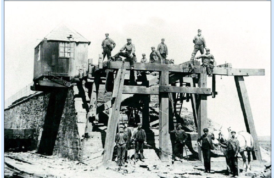
Workmen dismantling Bell Brother's Huntcliff Mine
